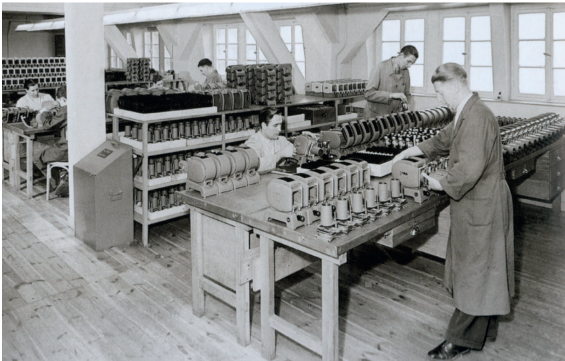
Final assembly of the 35 mm projektor in the topfloor of the Hausertor plant
