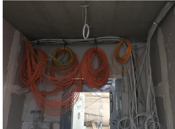
Rohinstallation Elektro
